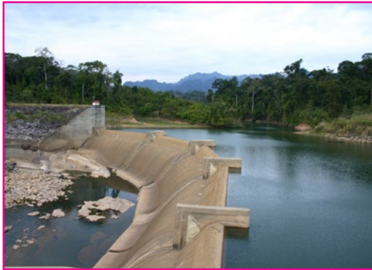
A section of the Theun-Hinboun Dam © Laurence McGrath, 2005 | Source: Wikimedia Commons.
